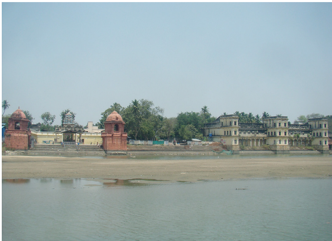
Fig. 2: Kalyana Mahal Chattram (extreme right) and other Maratha buildings on the bank of the Kaveri river, Tiruvaiyaru
